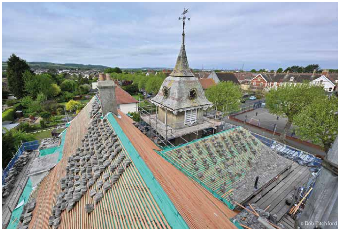
The roof of the Public Hall on 6th May.
