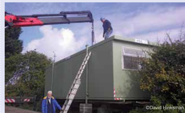
The arrival of the Portacabin at the green in May 2015
